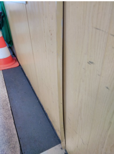
Container caisse : renforcement sol
