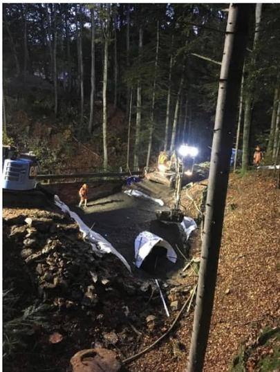
*Pose tube de gainage SYTEC*
